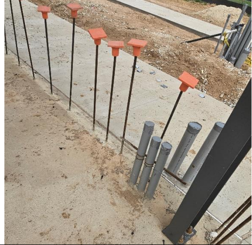
Electrical preparation for dugout
