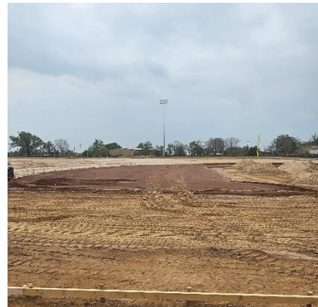
Base paths and framing for warning track between dugouts
