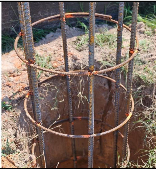
Bases for parking lot light poles ready to pour
