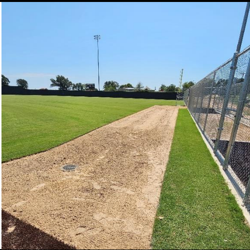
New sod to replace high traffic area from warning track installation
