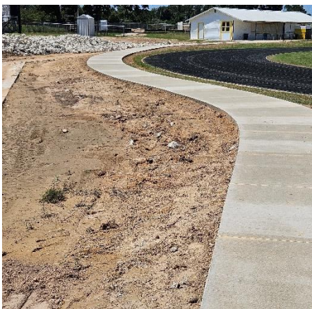
Endzone sidewalk will need re-grading and rip rap rock replaced
