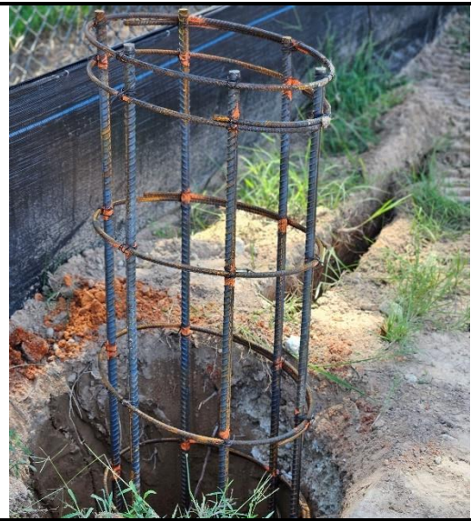
Bases for parking lot light pole
